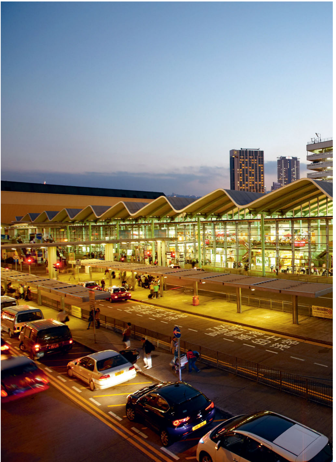
Mass Transit Railway (MTR) Hung Hom Station, Hongkong, China
